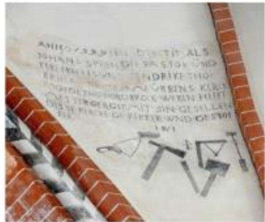
Figure 5. Text and tools restoration 1599. Church of Noordbroek, 1599.
