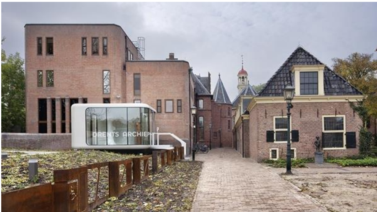
Image 14: the new entrance pavilion designed by Zecc Architects in 2012.
