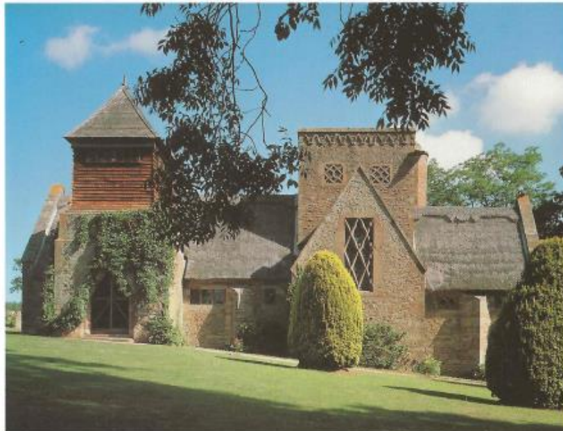
Appendix 44: William Richard Lethaby, Exterior of the All Saints Church, Brockhampton, Herefordshire, UK, 1901-1902.
